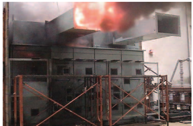
Arcing due to internal fault test
